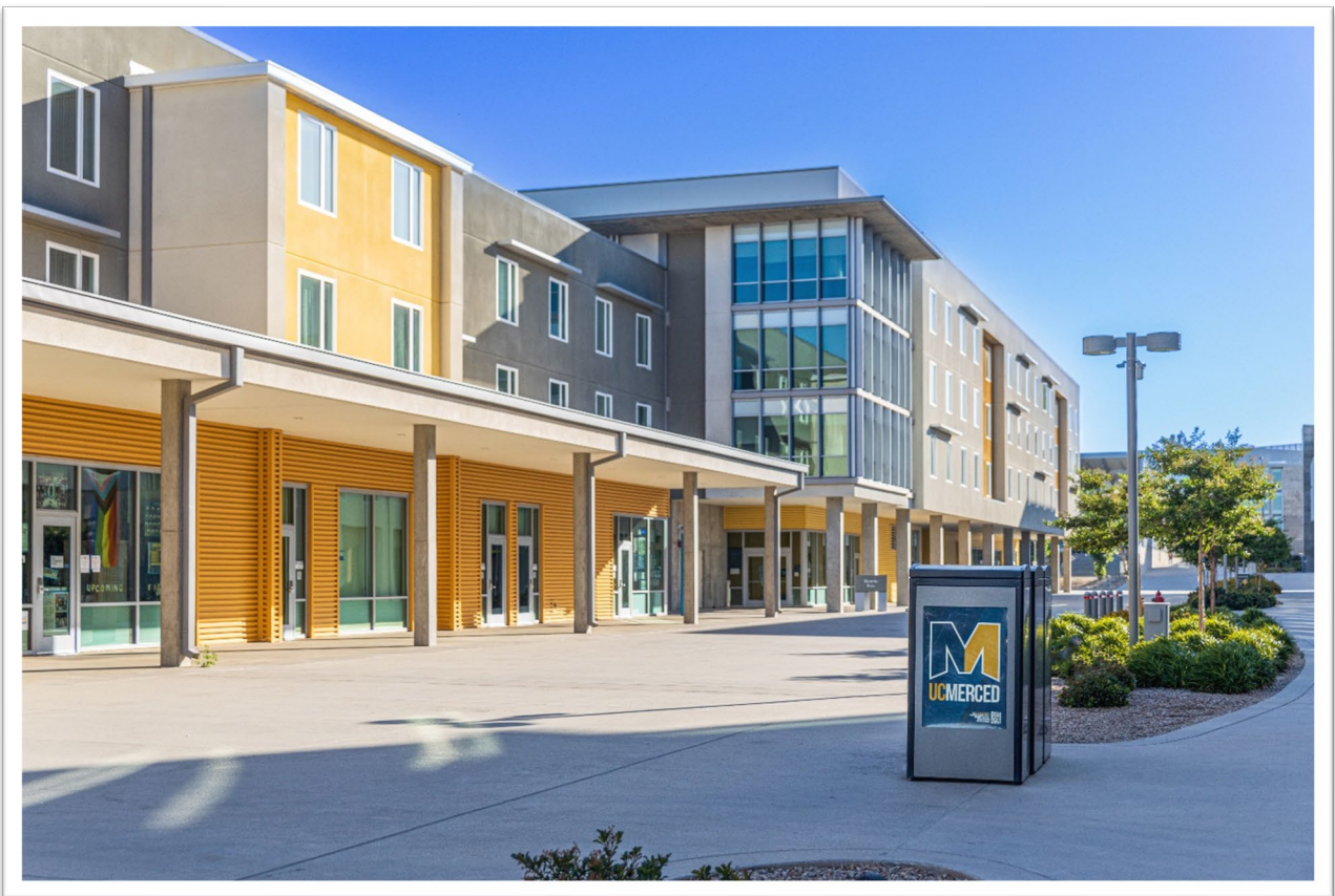
UC Merced Residential Facility
